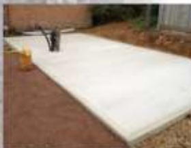
Concrete slab for plant room and pellet fuel store
