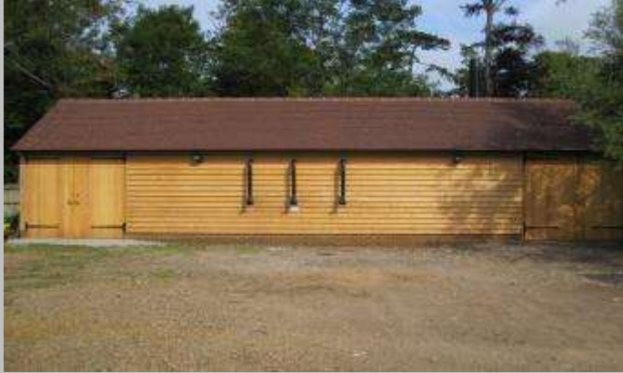
Purpose built plant and store
