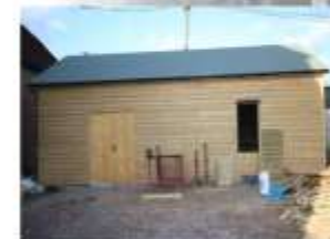
Plant room and pellet fuel store, designed and installed by Baystar
