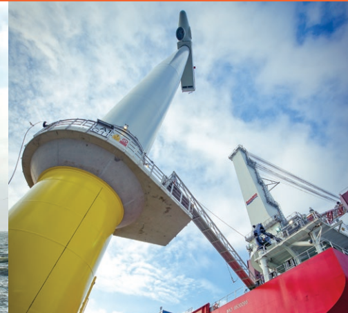
Final turbine installation, London Array, Thames Estuary.
