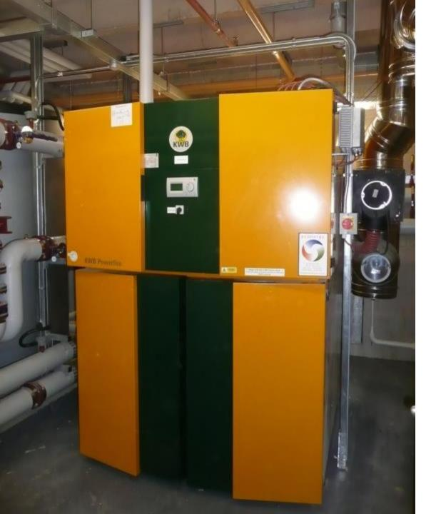
150kW wood pellet boiler installed in a Cheltenham school
